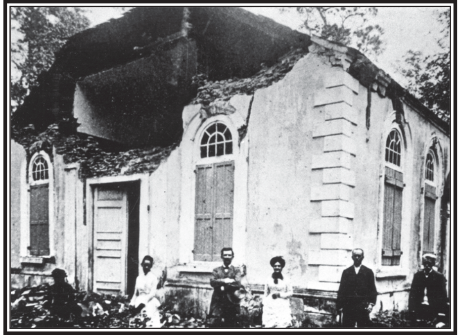
The Goose Creek Church in Charleston was damaged in the 1886 quake.
