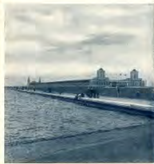
CHICAGO'S BEACH MUNICIPAL RECREATION PIER
