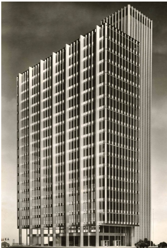
Circa 1954 rendering of the Inland Steel Building showing the service core of the building separated from the main volume. Credit: Ryerson and Burnham Libraries, Historic Architecture and Landscape Image Collection, c.1865-1973.
