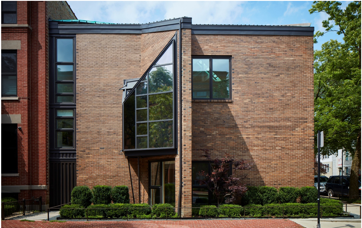
2022. Changes to the exterior include the addition of a cantilevered bay window and an expanded vertical window on the Eugenie Street elevation. These were designed by Netsch around 1990 and are significant.
