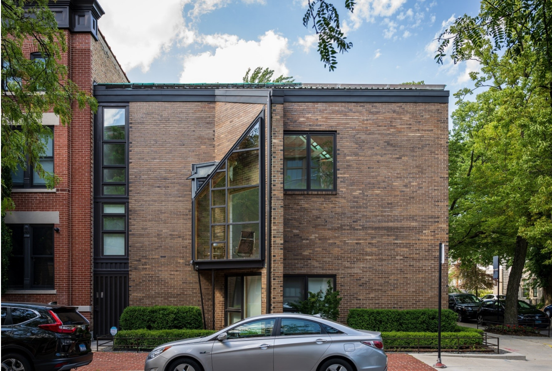
The south elevation of the Clark-Netsch House with its sharply angled bay.
