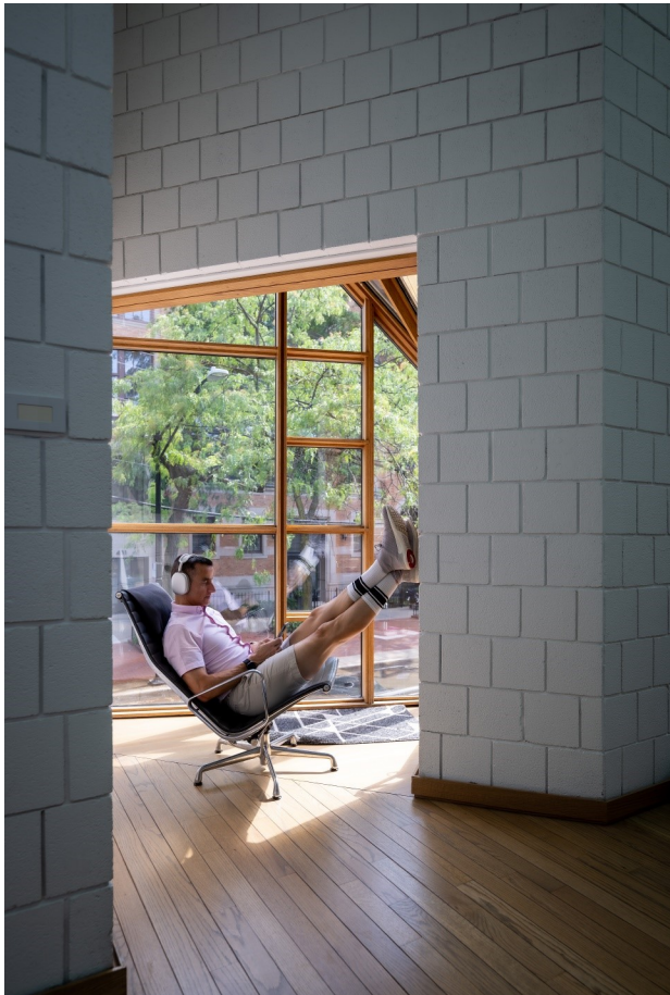
A sunny alcove was added to the house by Netsch around 1989. The walls are concrete block.
