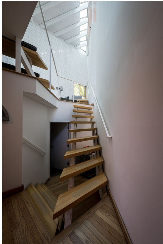
Open riser stairs access the multiple split levels of the interior.
