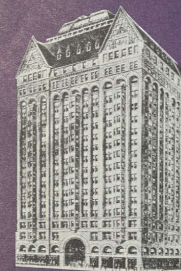
From 1894 to 1899 the law school was located on the seventh floor of the Masonic Temple located on the northeast corner of State and Randolph.
