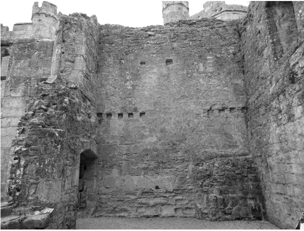
Fig. 3.38: Floor joists with gap for trimmer and faint scar in surviving plaster for staircase from ground floor against the external northern wall of the kitchen. Note the rebuilt oven below. Photo by Penny Copeland.
