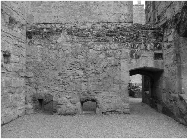
Fig. 3.15: Southern cross wall of western range showing relieving arch and flue or stoke holes. A further retaining arch is visible on the northern side. Note knife sharpening effect on doorway. Photo by Penny Copeland.
