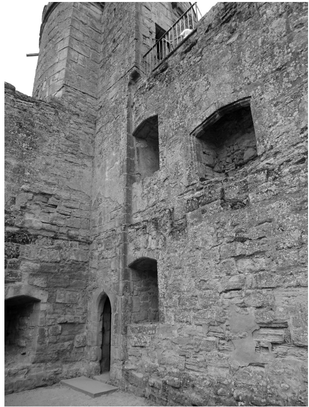
Fig. 3.30: Possible straight joint between north-west tower and north wall. Photo by Penny Copeland.
