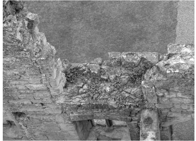
Fig. 3.34: View down only narrow window jamb to west, and rebated door jamb to right. The door jamb sits slightly over the triple door wall at the end of the Great Hall. Photo by Penny Copeland.
