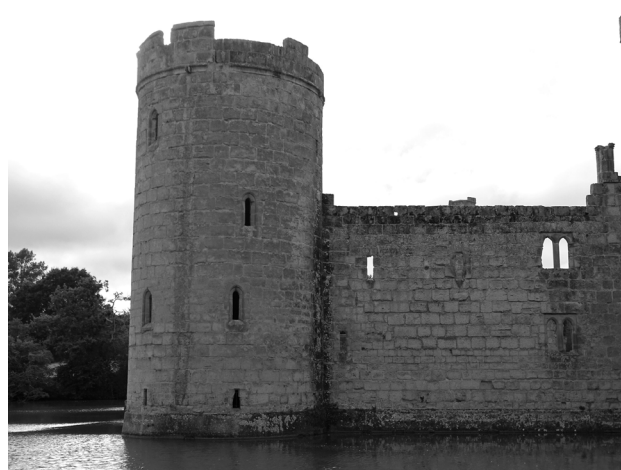
Fig. 3.31: Southern section of the east curtain wall showing different building seasons. Photo by Penny Copeland.
