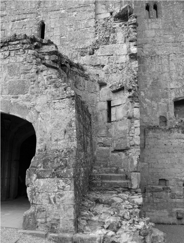
Fig. 3.14: Buttress against gatehouse, built up against stair to reach chamber. Photo by Penny Copeland.
