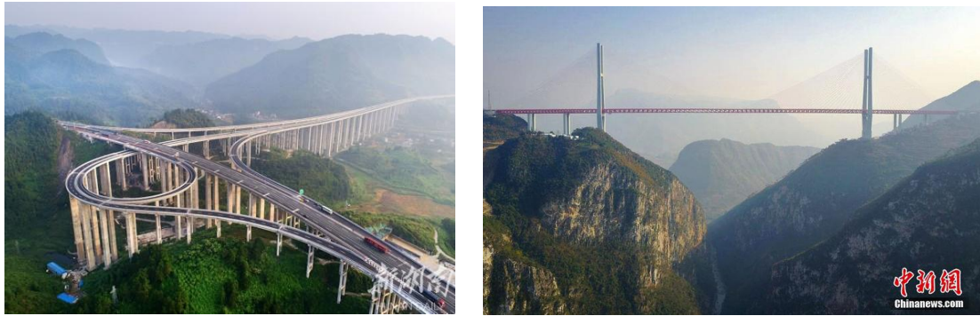
Figure 11 Shijiazhai Interchange on the Yongji Highway in western Hunan, Middle Yangtze and the world's highest bridge of Duge Beipanjiang Bridge in Guizhou (565m deck height, 720m span (source: Hunan daily, 2017. chinanews.com).
